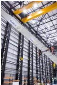
ORE Catapult Marine Test Site; Blade Test; Powertrain facilities; CPTC Energy Link Lab; HV Lab
